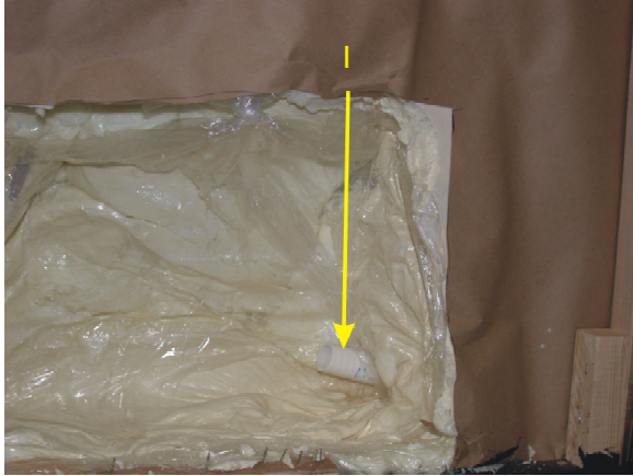
I. Electrical Conduit Before Trimming
